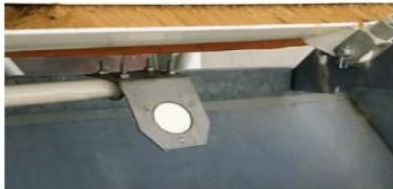
Sensor installed in material chute under silo outlet
